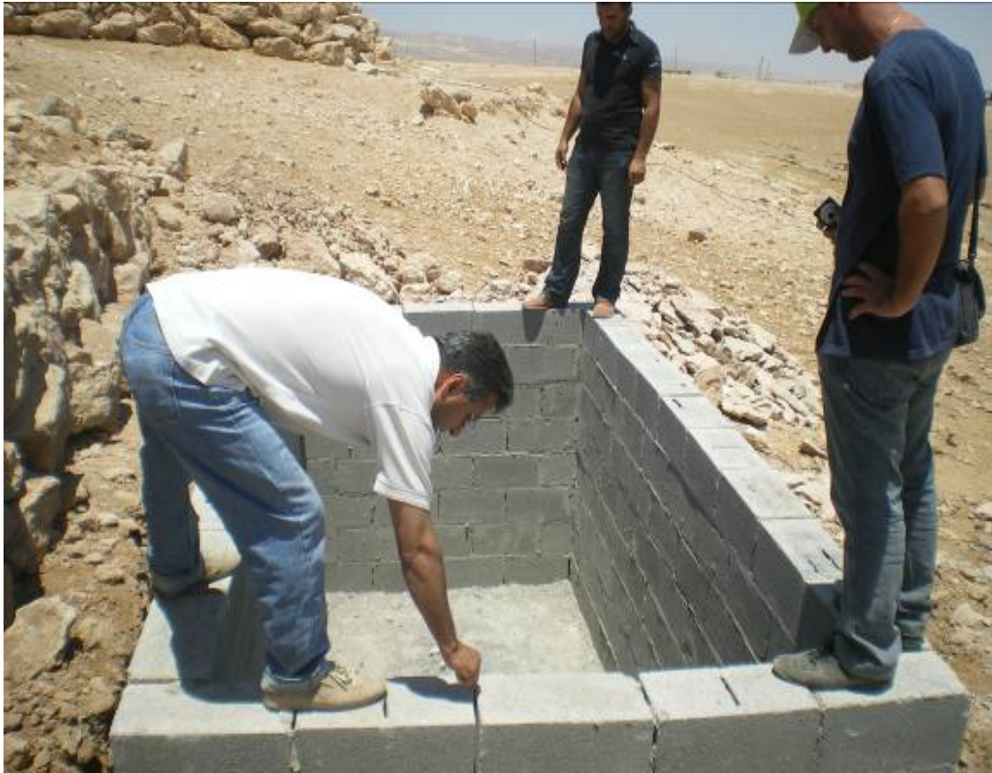
Photo (7), GWWT unit under construction at Az Zuweidin
