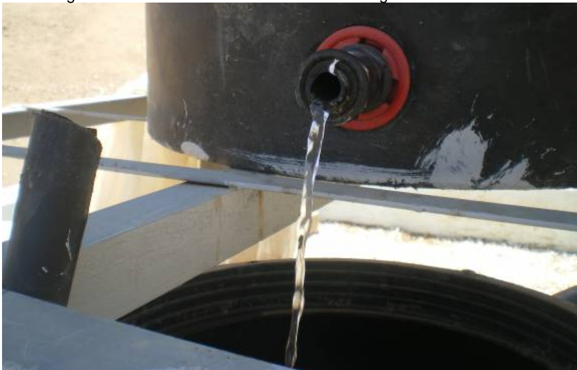
Photo (9), Treated gray wastewater flow to the irrigation system at An najada.
