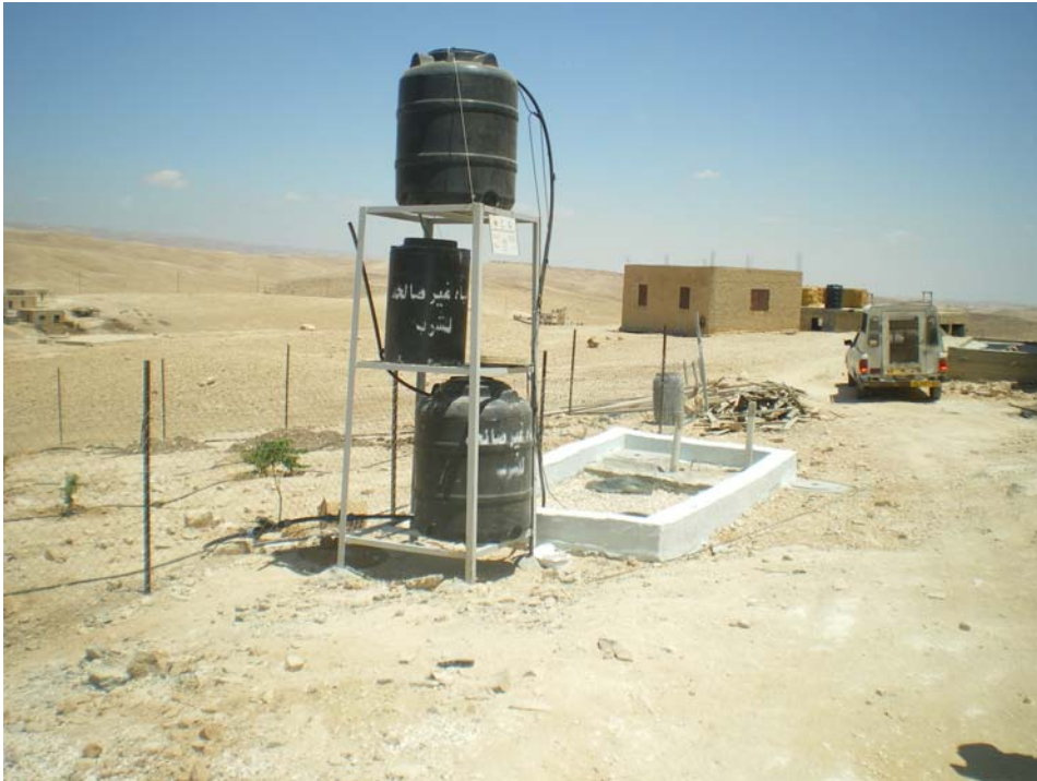
Photo (5):- A completed GWWT unit at An Najada.
